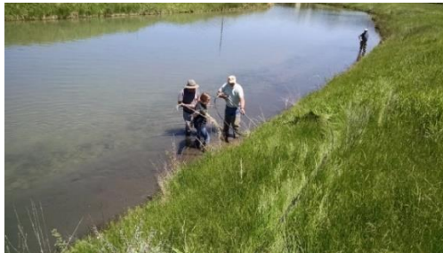
Matt, Duane and Lilly using water-jet to create hole for the willow cutting.
