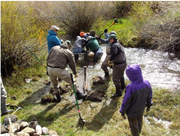
Securing logs with rebar.
