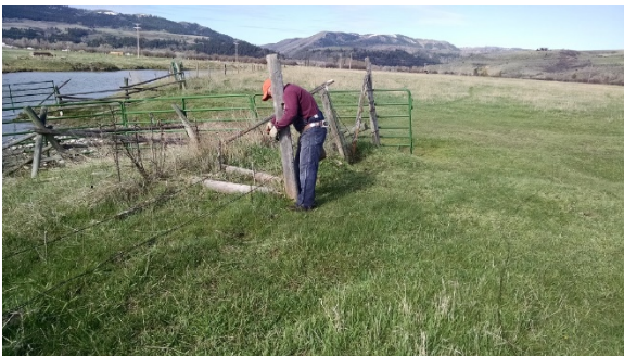
Rory, removing the old wire.
