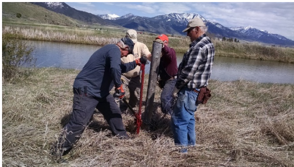
Rob, Scott, Rory and Bill pulling a wood fence post with a little assistance from a handyman jack.
