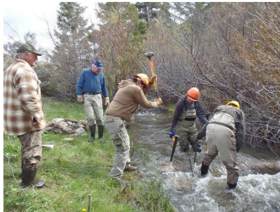
Pounding re-bar to secure log structure.
