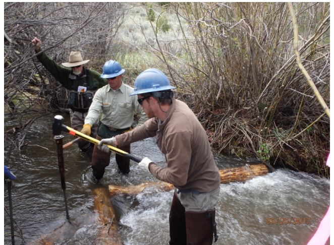
Jerry, Jay and Nate secure the structure with rebar.
