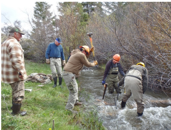
Pounding re-bar to secure log structure.
